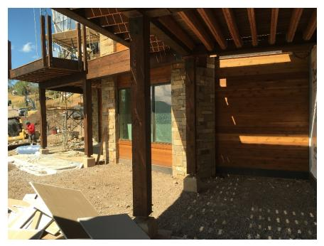
8 x 8 timber posts – stained board form concrete piers 18" x 18"
