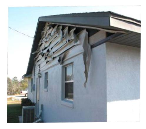
**Defensible Space?** It takes 5 sec to produce second degree burns under same conditions it takes 27 mins to ignite a wood wall (16 Kw/m2)
