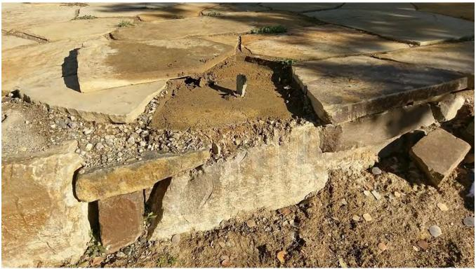
No concrete structure beneath the sand-set flagstone patio in the GE
