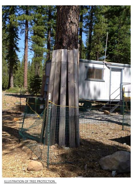
NOTE: ALL TREES TO REMAIN WITHIN THE LIMITS OF CONSTRUCTION SHALL BE PROTECTED AS ILLUSTRATED ABOVE.
