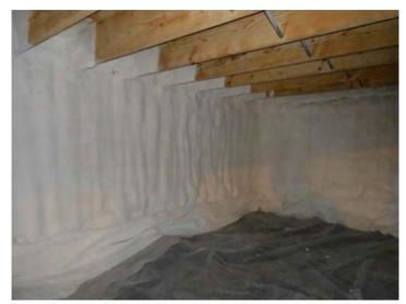
**Outstanding Insulation/Air sealing in Crawl Space**
