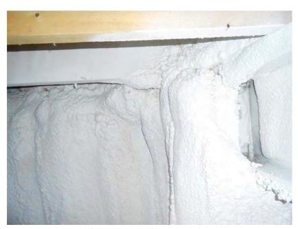
**Typical Spray Foam Insulation in Crawlspace**
